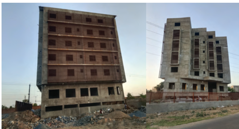
Ongoing Construction of an Educational Building
